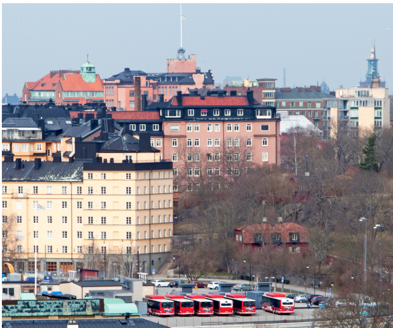
Biogas buses parked at the bus depot below Henriksdal. The fueling station is connected directly to the Scandinavian Biogas plant at the top of the hill.
